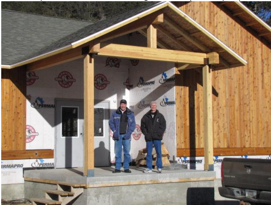
The front porch and new wood siding on a sunny January day...
